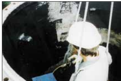
WEICON WR - Coating of a CO 2 cleaning installation
